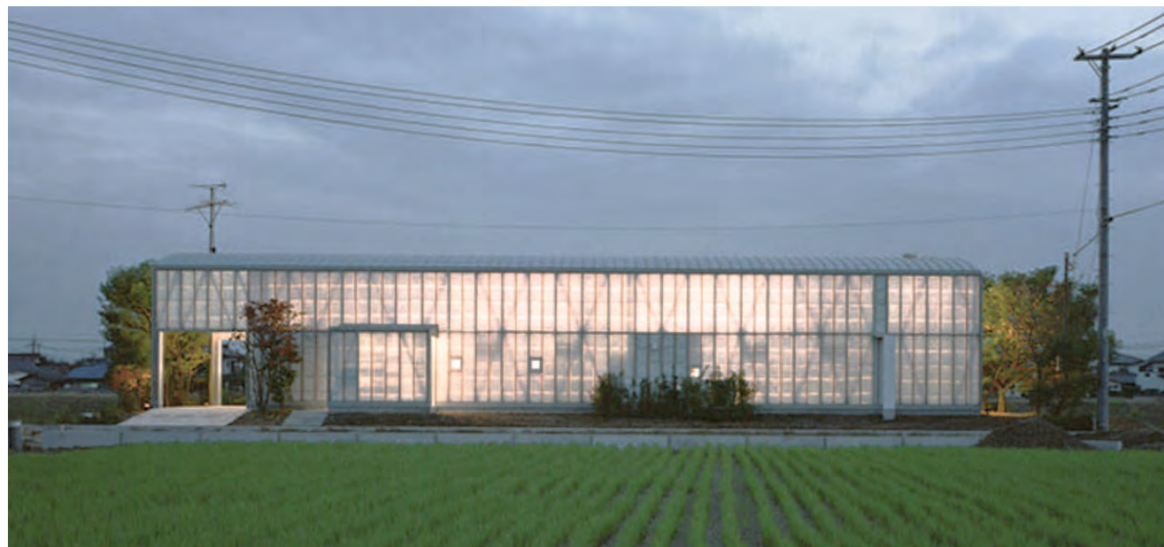
Light passes through the translucent skin, making the building read as a glowing lantern from the exterior. Behind the skin, the diagonal cross-bracing is faintly expressed, exposing the lateral stability system and giving the façade a clear structural order.
