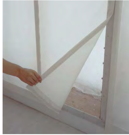
Removable Velcroed Nylon Fabric Membrane as an Internal Translucent Skin
